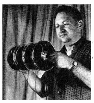
Today, tapes can be bought in (left to right) standard-length, extra-play, double-play, and triple-play sizes. Extra footage is put on a 7-inch reel by cutting thickness of tape base, and, for triple-play, by reducing the thickness of the oxide coating.
