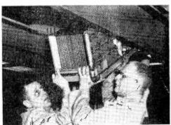
Solid-state air conditioner is being installed in existing air duct (top right). Complete unit is shown upper left with solid-state section located in middle. Diagram at left shows how room and outside air are mixed and cooled. Only fan blower and damper move.
